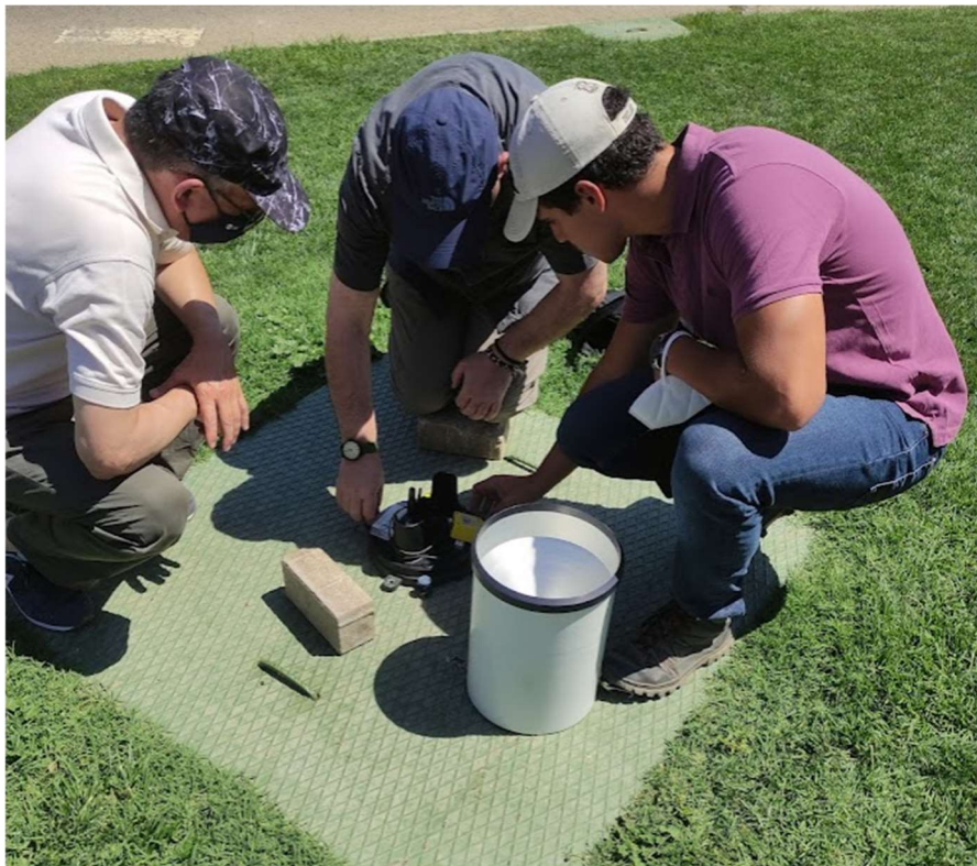
Figure 17. Rain gauge installation and leveling
