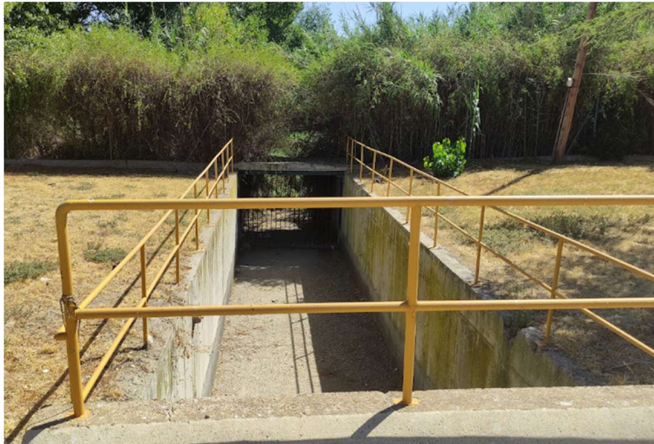
Figure 16. By-pass channel from the primary treatment to the river
