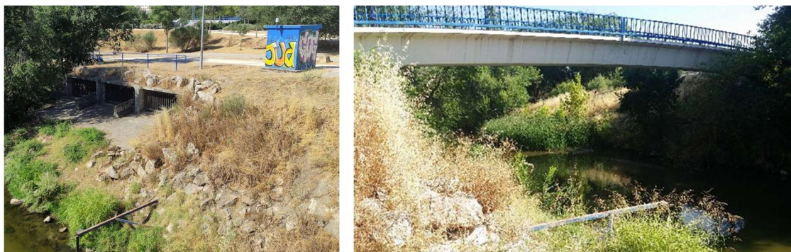
Figure 22. General view of the monitoring point with the Oliva tank CSO discharges and the monitoring stand in blue.
