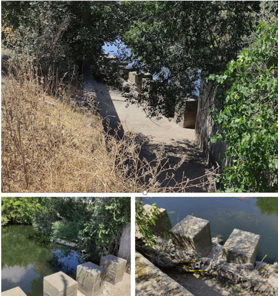
Figure 26. Installation point A upstream Sur WWTP by-pass
