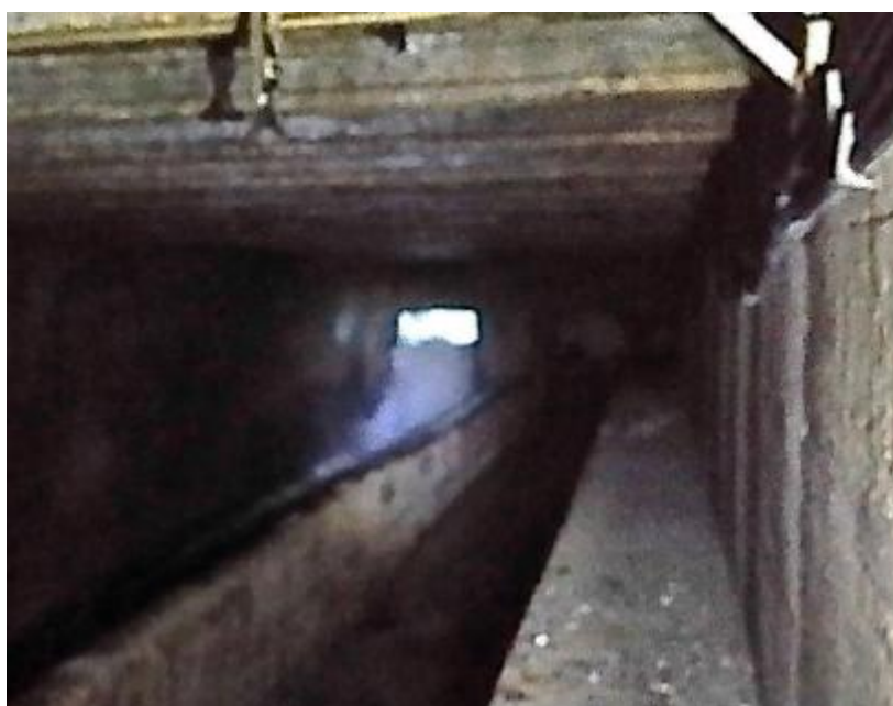
Figure 22.- Weir chamber from the left margin interceptor (right channel) with the wall weir and the window are the flows coming from La Gavia WWTP. When the water level in the left margin interceptor raises above the wall these flows join the ones from La Gavia and are discharged in the river.
