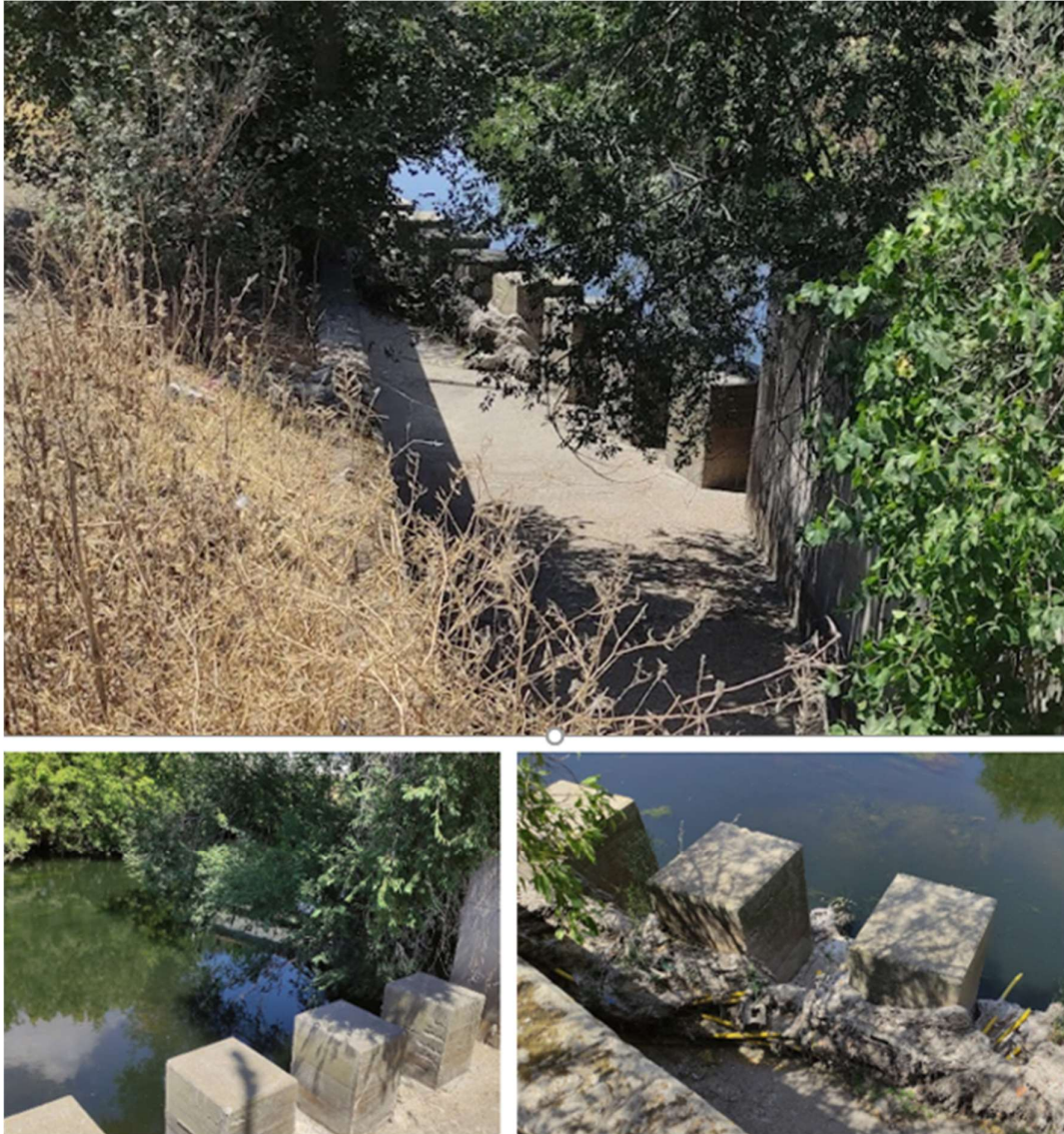
Figure 26. Installation point A upstream Sur WWTP by-pass
