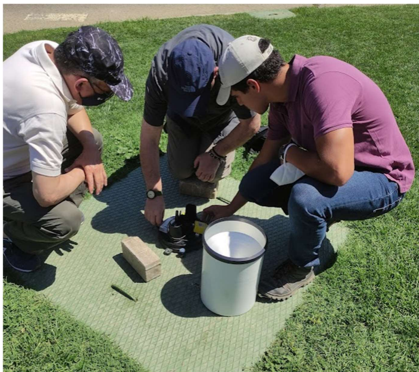
Figure 17. Rain gauge installation and leveling
