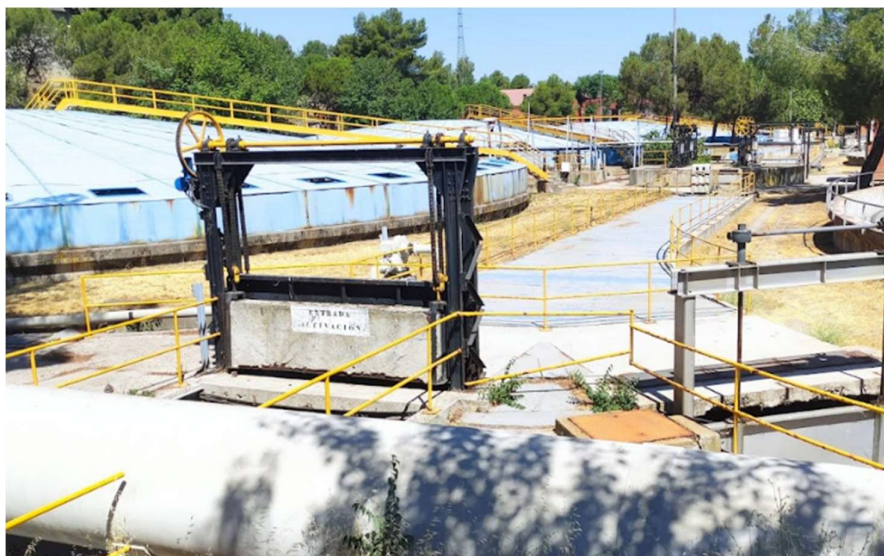
Figure 15. Water channel driving the waters from the primary to the secondary treatment. At the left waters are driven to the secondary while whenever the biological capacity is surpassed the waters are driven right to the river.
